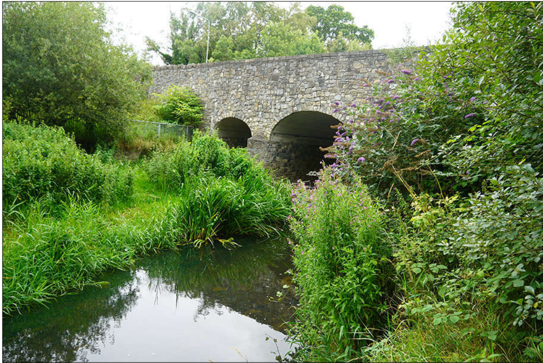
Plate 12-9 Kildare bridge, from SE.
